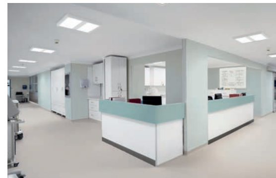
Reception and waiting areas: Perfect light thanks to UGR < 19 and PC diffusor.
